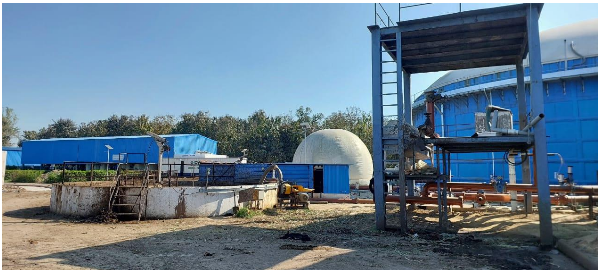
Fig 1 & 2: Glimpses of the Bio Gas Plant
