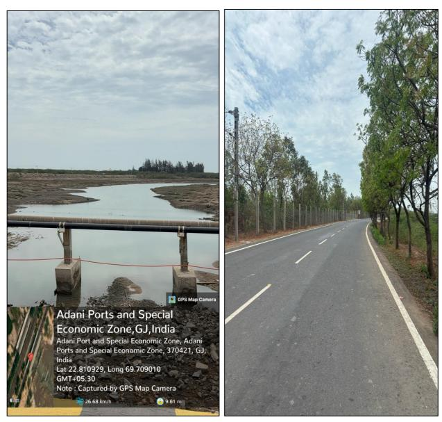
Figure 2-11: Minor Stream Crossing in NG Pipeline Network
