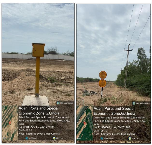
Figure 2-9: Cathodic Protection Device/Rectifier in Pipeline Network
