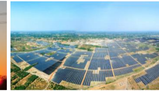
648 MW Ultra Mega Solar Power Plant
