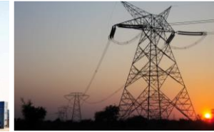
Longest Private HVDC Line in Asia
