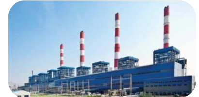
Largest Private Thermal Power Station in India
