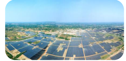
648 MW Ultra Mega Solar Power Plant
