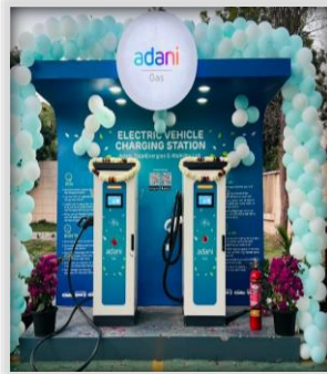
Lucknow Airport, Uttar Pradesh
