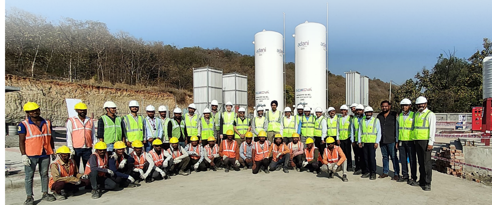
▲ Safe installation and commissioning of LCNG plant at Lunawada (Kheda GA)
